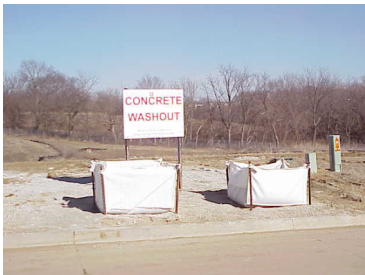
Waterproof bags used for containment of washout wastes.
