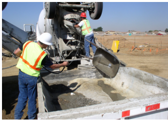
Roll-off used for containment of washout wastes.
