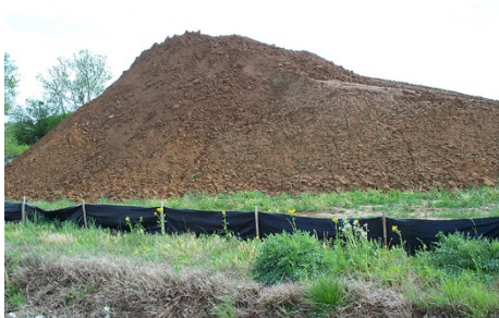
Silt fence around soil stockpile. Photo credit: Barry Tinning, Tetra Tech
