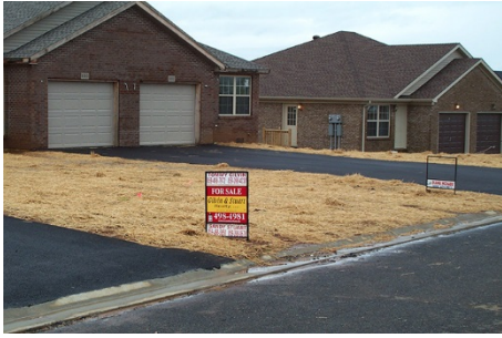
Straw mulch can be used to both prevent erosion and minimize dust from a site. Photo credit: Barry Toning, Tetra Tech.
